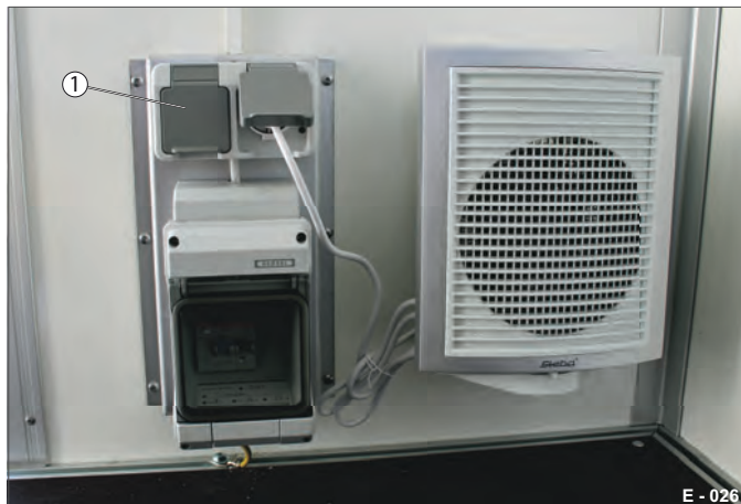
Fig. 8 Distributor box with sockets
