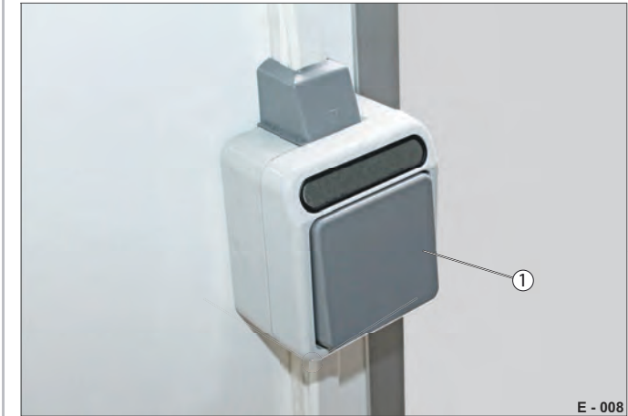
Fig. 7 Light switch for 12 V and 230 V
