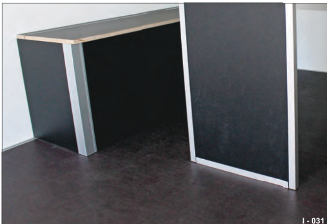
Fig. 3 Floor (18 mm thick) made from multi-layer wooden plates
