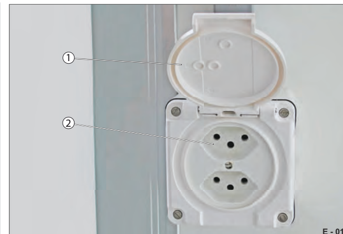
Fig. 16 Twin sockets
