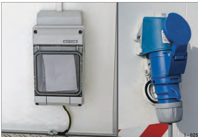
Fig. 19 230 V power supply
