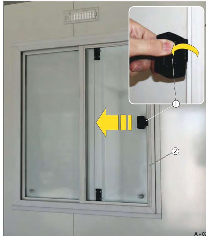
Fig. 5 Opening the sliding window
